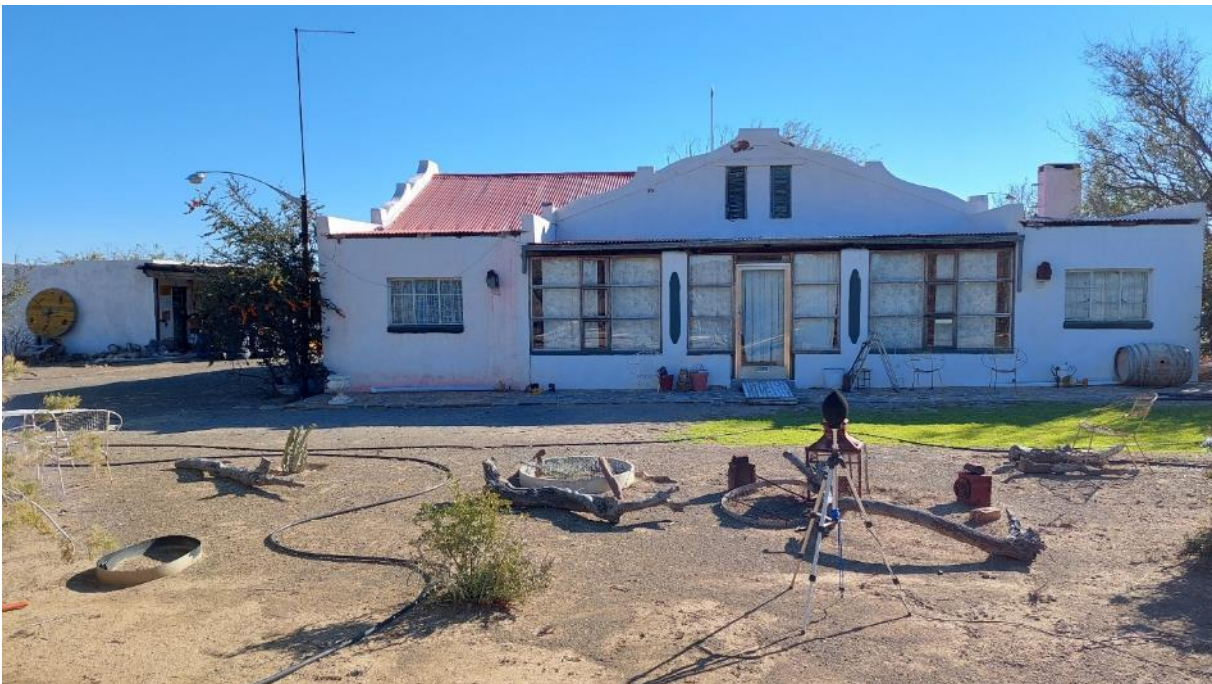
Photos E.1: Measurement location at SGEKLTSL01
