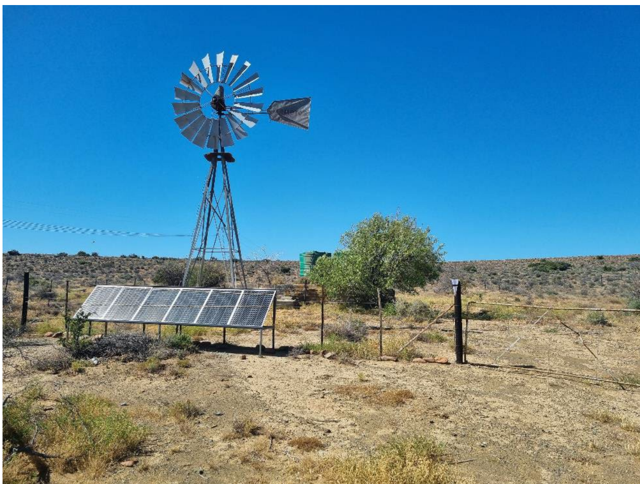
Figure 2: Borehole with water trough
