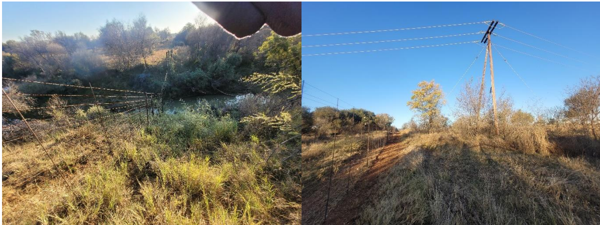
Figure 6-1 Impacts observed during the assessment included existing fences and powerlines.
