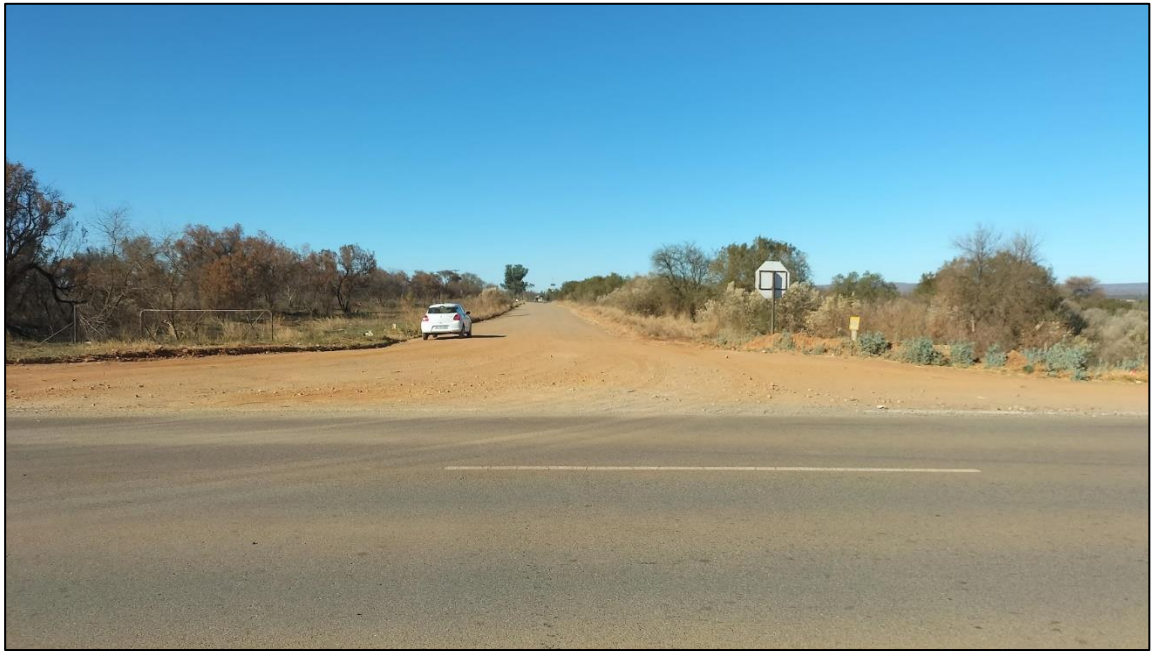
View of gravel site access road at its intersection with D114.
