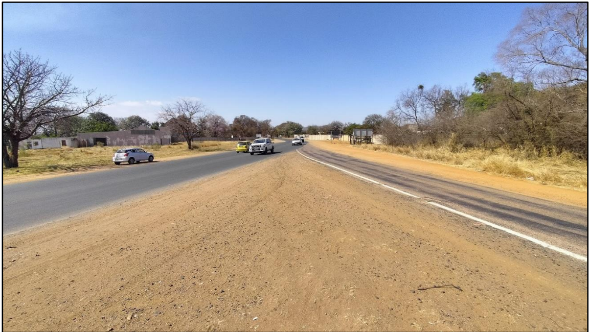
View along R565 towards Boshhoek from D114/R565 intersection
