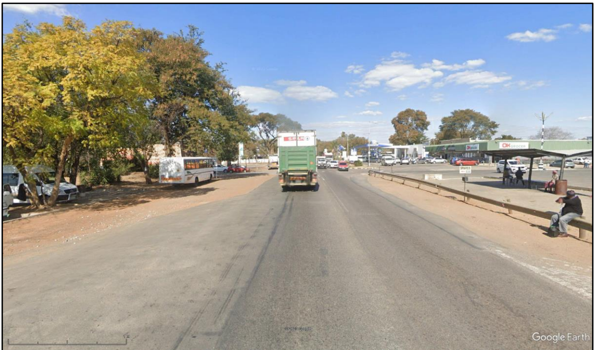
Taxis were noted stopped alongside R565 alongside the guardrail (should be stopped in the roofed taxi loading area). The main delay was due to a right-turn vehicle (i.e. movement as shown in image below) and taxi stopped alongside thus preventing vehicles bypassing the right-turn vehicle.
