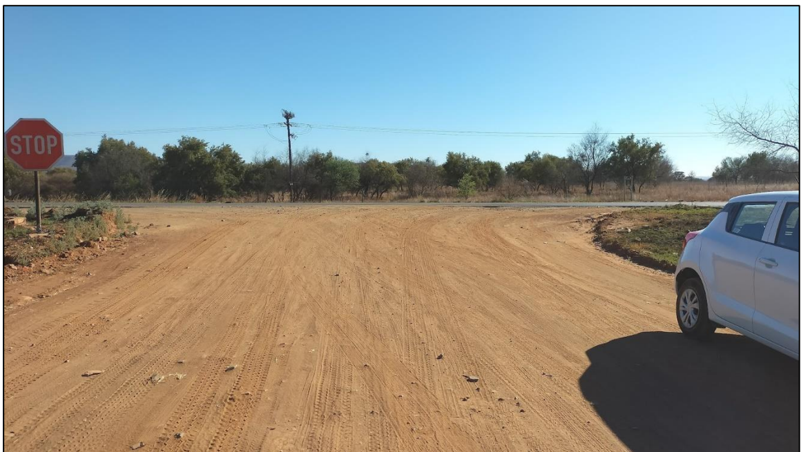
View of gravel site access road approach to D114 (Priority control road signage in place)
