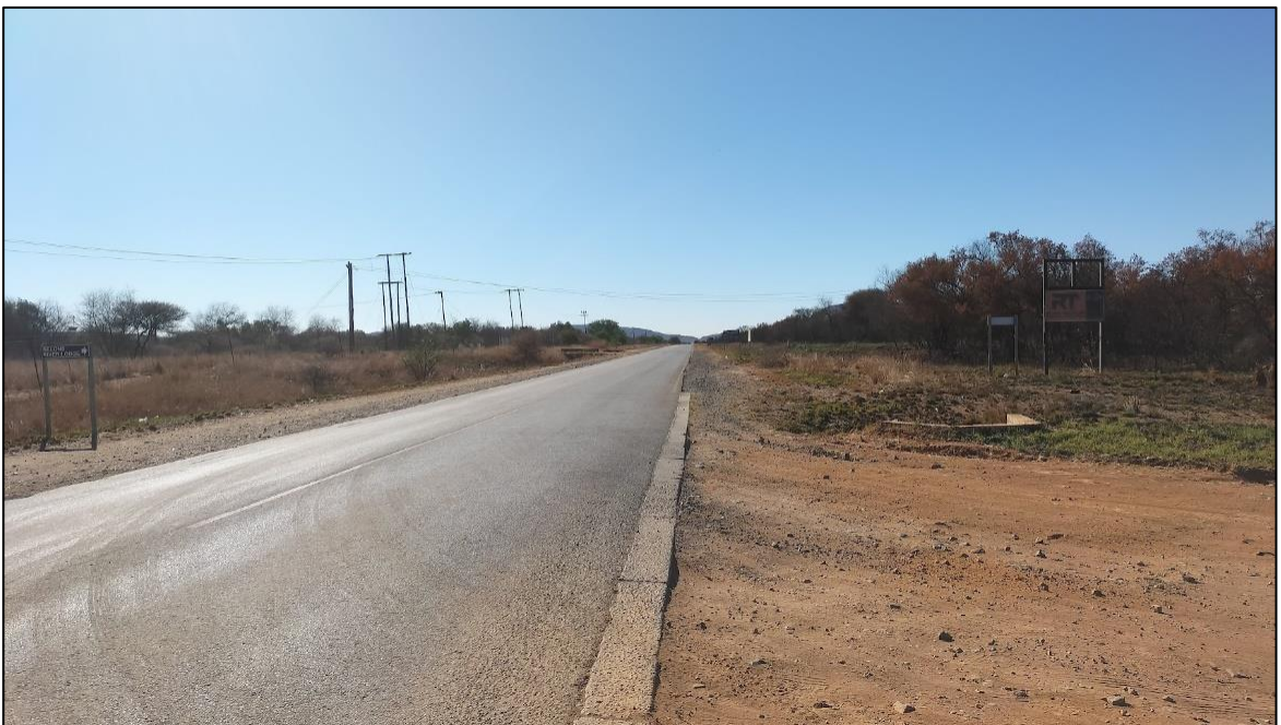
View to right of gravel site access road intersection with D114. Note concrete edge beam.
