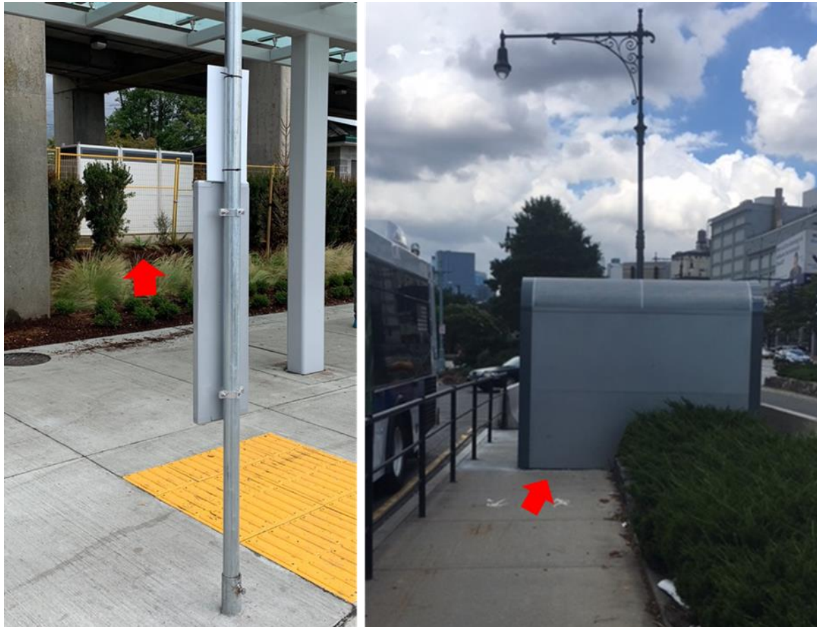
Figure B-6 450 kW In-route Charger Power Modules
