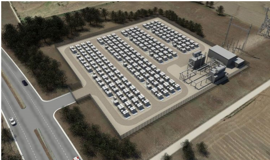
FIGURE 7-6 SOLARCITY'S TESLA BATTERY STORAGE FACILITY, HAWAII
