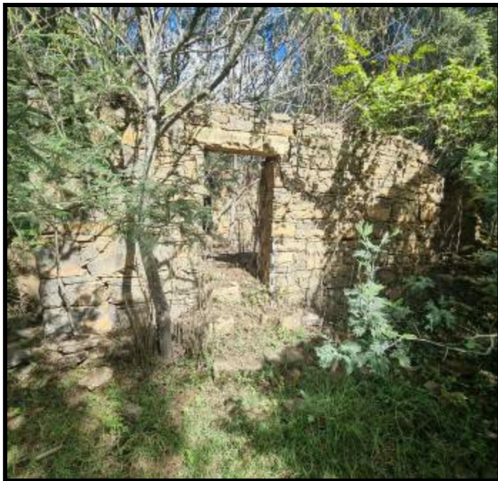
FIG. 13: BUILT STRUCTURES AT ROCH05
