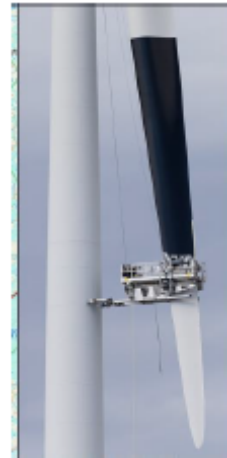
Figure 1: The single black-blade in the process of being painted in situ, at the Smøla Wind Farm. Painting white blades black after they are erected is more expensive than producing them at source.
