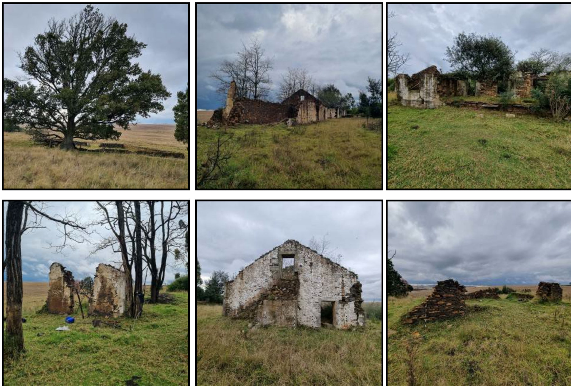
FIG. 45: BUILDINGS AT TL03 (WELTEVREDE)
