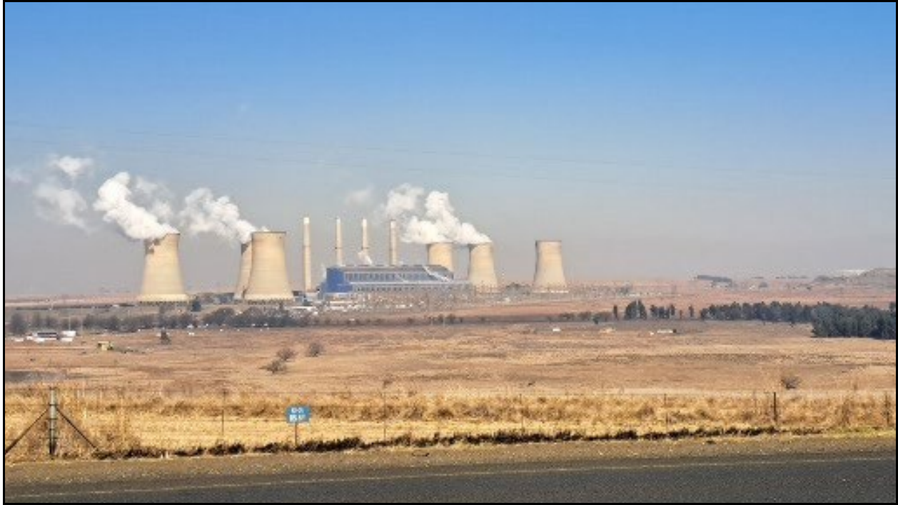
Photograph 3.2: Camden Power Station
