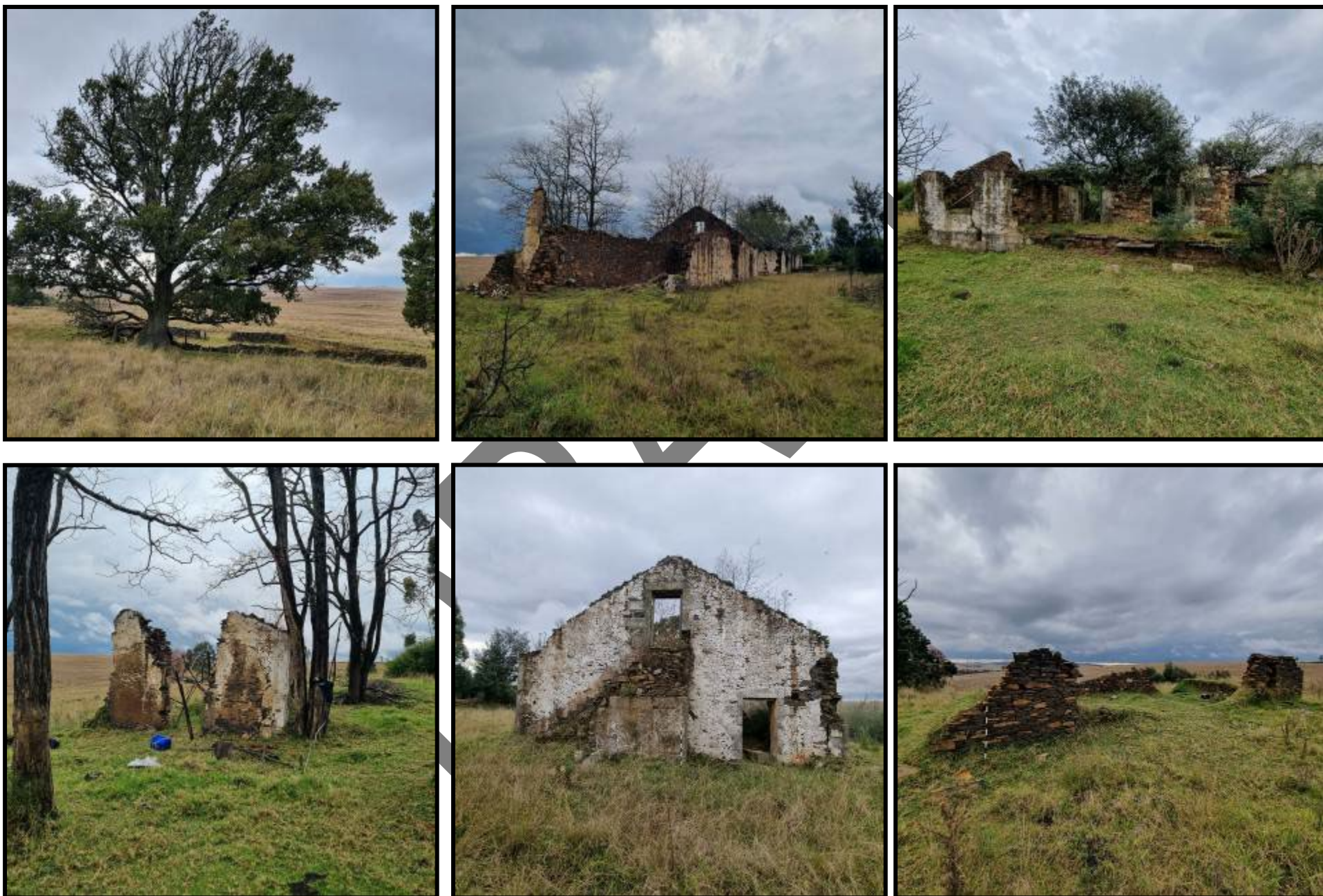
FIG. 53: BUILDINGS AT TL03 (WELTEVREDE)
