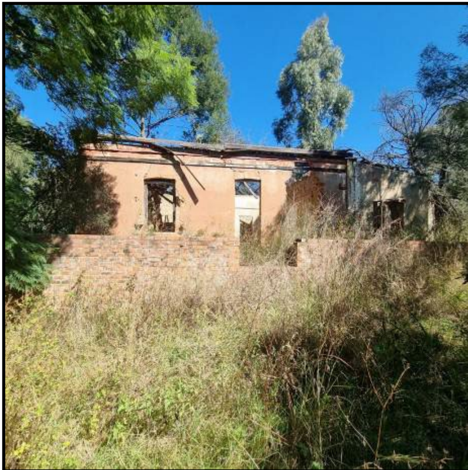
FIG. 14: BUILDING AT EMVE05
