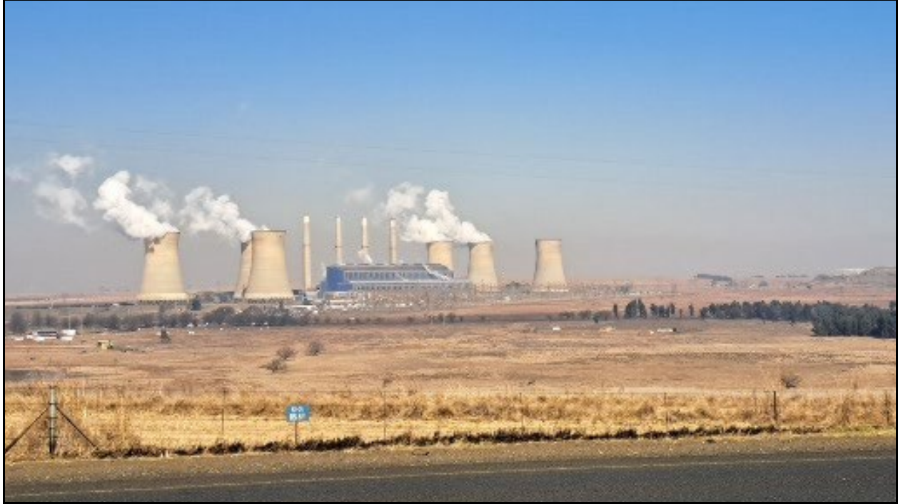
Photograph 3.2: Camden Power Station
