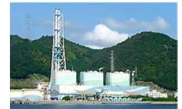
Mix combustion in coal fired boiler
