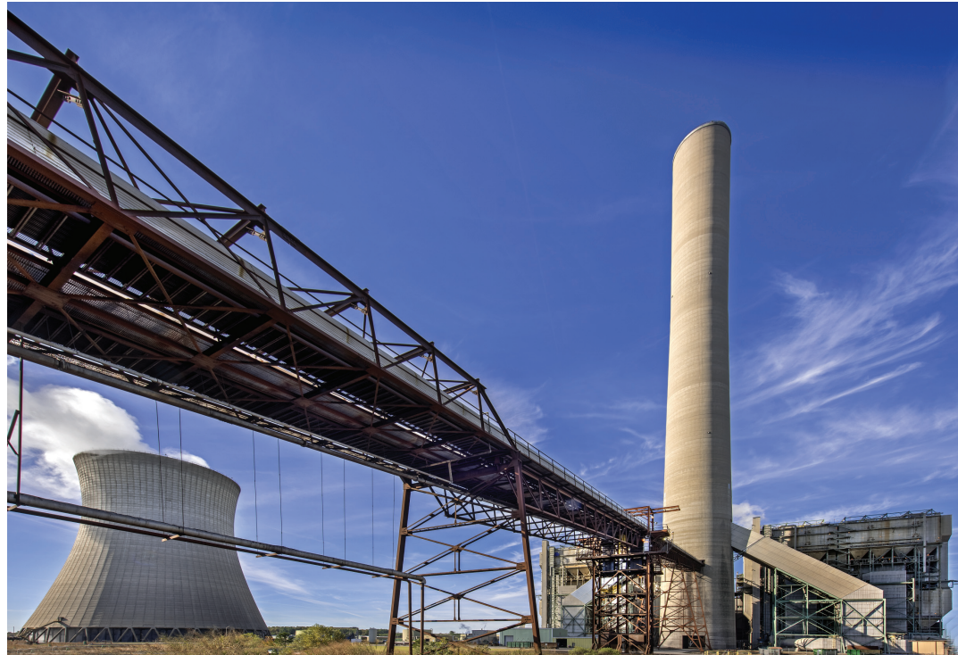
In meeting the April 2016 compliance requirement of EPA's MATS Rule, Entergy significantly reduced mercury emission levels at its Independence, Nelson 6, and White Bluff (pictured) coal facilities by installing mercury emission controls that use activated carbon injection.
